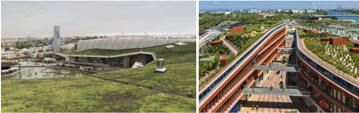
Figure 2 & 3: Extensive GR on Lagoh shopping center and intensive GR on TORRE Sevilla . Retrieved from ZinCo Cubiertas Ecológicas S.L. (2019) and Sevilla21, (2023).
